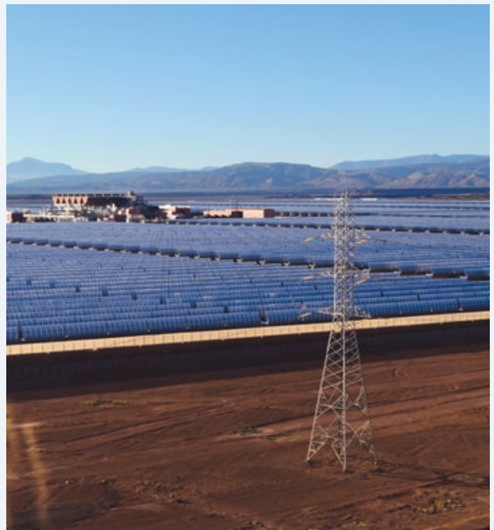
NOOR solar complex project in Ouarzazate, Morocco. African Development Bank Projects photo Collection.
