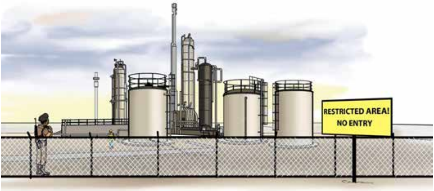
A central processing facility where the mixture of oil, gas and water is separated
